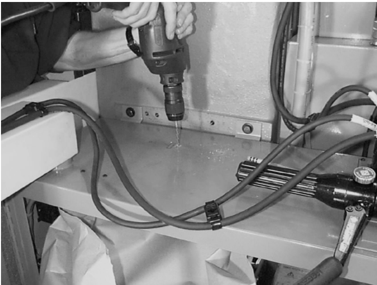
Figure 11-93 Drill Starting Holes
