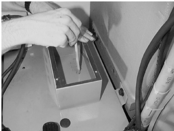
Figure 11-90 Mark Positions to be Drilled Out
